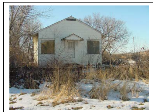
Figure 14: Boarded up House & Overgrown Vegetation
