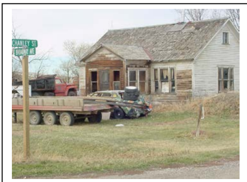
Figure 13: Deteriorated Residence & Abandoned Cars
